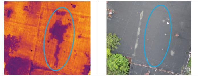
Potential Roof Leak - Temperature variance in IR, no visible water on roof
