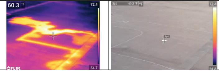
Irregular thermal pattern on otherwise uniform roof surface. Closer inspection of irregular area revealed a small slit in the roof membrane.
