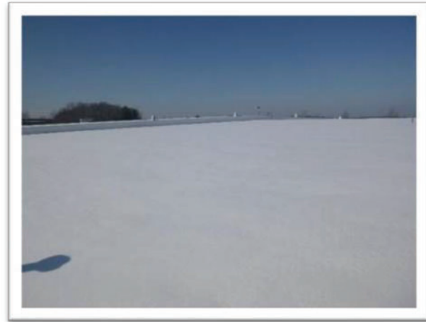
Photo #2 Flat roof proposed for solar PV
