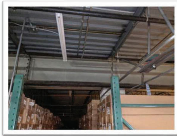
Photo #4 21-inch deep girders
